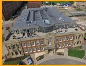
SINGLE PLY ROOFING
