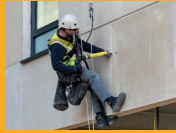
JOINT SEALING
