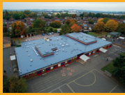
LIQUID APPLIED ROOFING
