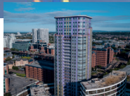
CONCRETE REPAIR (REFURBISHMENT)
