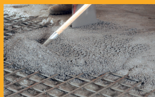
CONCRETE AND REPAIR
