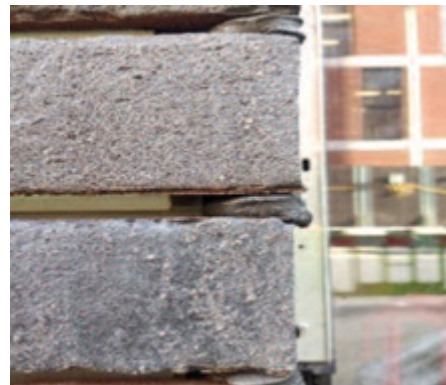
Photo 5 Correct complete bead around corner
