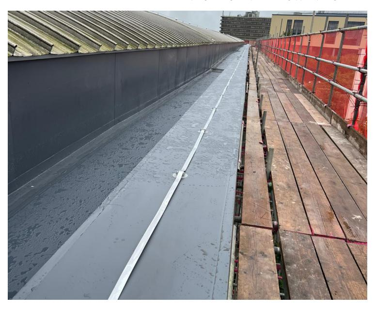
The Sikaplan® SGK-15 is a polymeric membrane based on premium quality polyvinyl chloride (PVC) with an inlay of glass non-woven and polyester fleece backing according to EN 13956.
