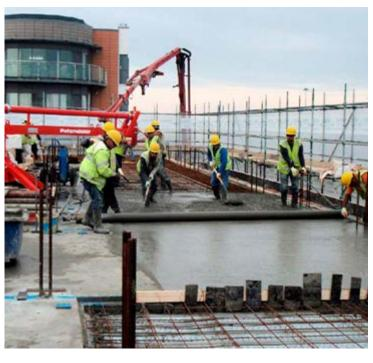
With the building now out of the ground, the car park is completely dry, with the watertight concrete providing a protective watertight shell. BBA approved Sika® Watertight Concrete works by incorporating two powerful admixtures that reduce the water content of the mix and in turn the amount of capillary pores, with a pore blocker to block the remaining pores.
