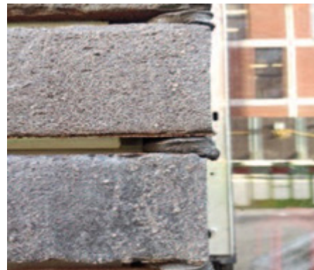
Photo 5 Correct complete bead around corner
