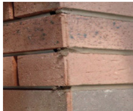
Photo 6 Incorrect mortar stops at the corner
