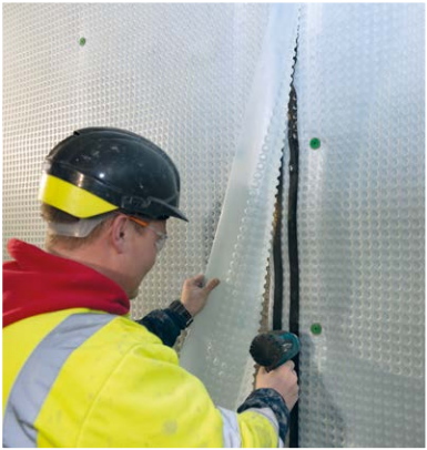
Sika cavity drainage system installation
