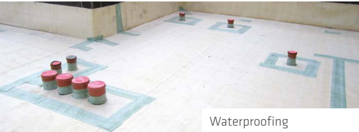
Joint sealing
