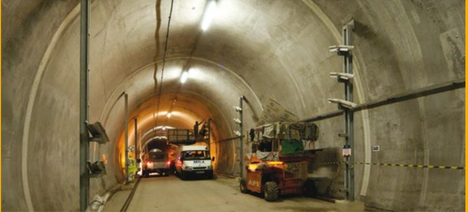
Before cables could be installed, the tunnel required substantial maintenance work including extensive waterproofing and structural repairs. A specialist Structural refurbishment specialist Stonbury with extensive experience within the water and power industries, was appointed to complete the application of a concrete repair and waterproofing system over a 16 week period.
