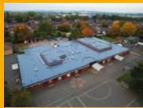
LIQUID APPLIED ROOFING
