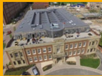
SINGLE PLY ROOFING
