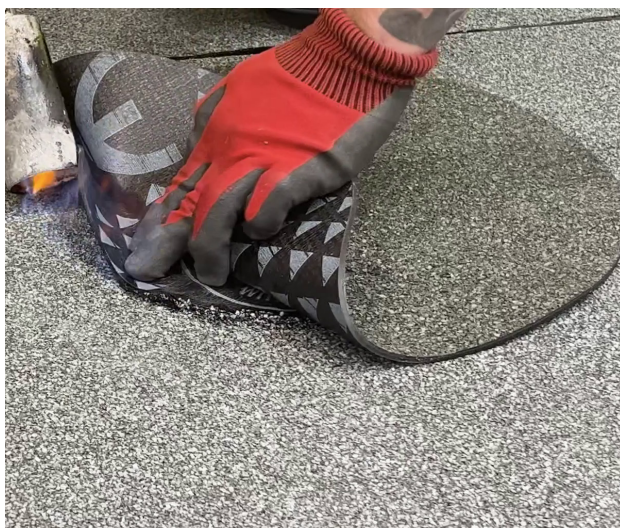
Torch application of the underlay.
