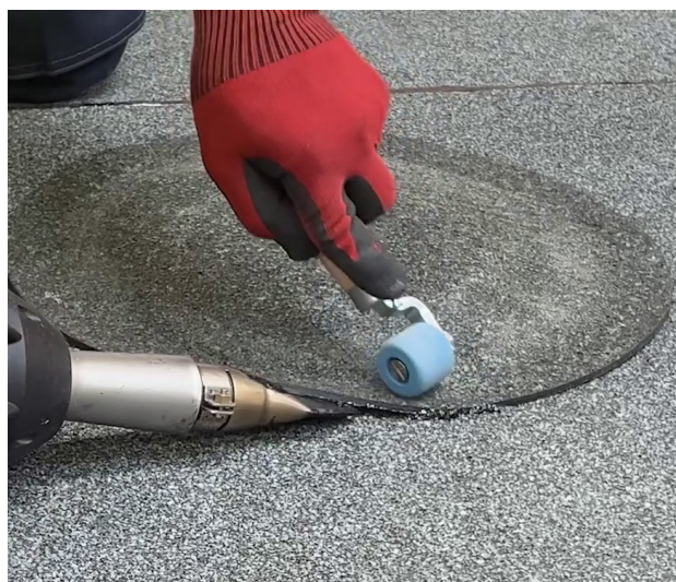
Hot-air application of the cap sheet.
