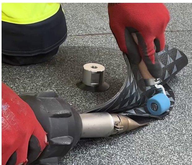
Hot-air application of the underlay.
