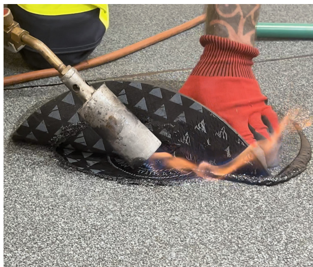
Torch application of the cap sheet.
