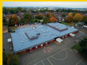
LIQUID APPLIED ROOFING
