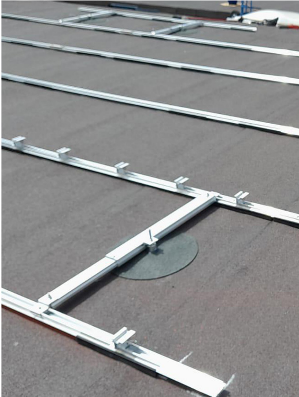
Installation of SikaShield® Anchors and Solar Mounting System.
