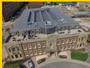
SINGLE PLY ROOFING
