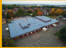
LIQUID APPLIED ROOFING
