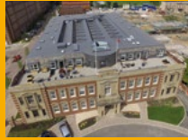
SINGLE PLY ROOFING
