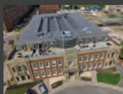
SINGLE PLY ROOFING
