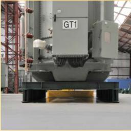
Alongside the textured floor that Sikafloor®-263SL offered, its durability is of the utmost importance to the solution. Should the concrete begin to fail under the weight of storage items, there is a risk that the air-beds of the Movetech air-skates will be damaged, rendering the expensive equipment inoperational. Sikafloor®-263SL can tolerate the most arduous usage – which combined with its smoothness, made it the ideal specification for the unusual project.
