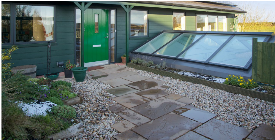
The roof garden constructed over a Sika Sarnafil green roof
