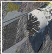
TBM heading injection
