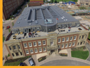
SINGLE PLY ROOFING
