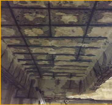
cleaning the areas in preparation for the application of Sika's reinforcement system. Firstly, the steel reinforcement was applied with <u>Sika® MonoTop®-610</u>, a high-performance, one-component, cementitious polymer-modified protection coating.
