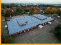
LIQUID APPLIED ROOFING
