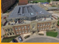
SINGLE PLY ROOFING
