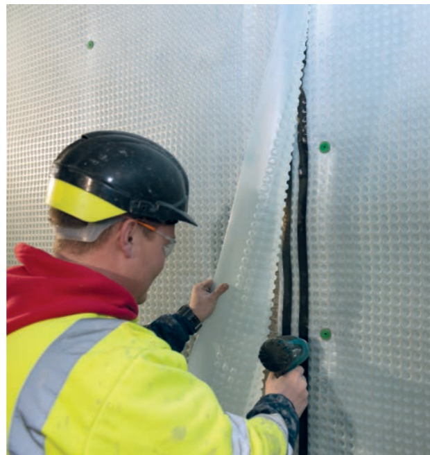
SIKA CAVITY DRAINAGE SYSTEM INSTALLATION
