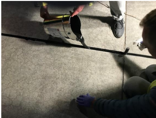
Picture 3: Application of Sikaflex-406 KC directly out of the pail
