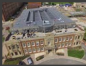
SINGLE PLY ROOFING
