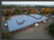
LIQUID APPLIED ROOFING
