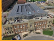
SINGLE PLY ROOFING
