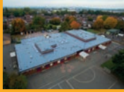
LIQUID APPLIED ROOFING
