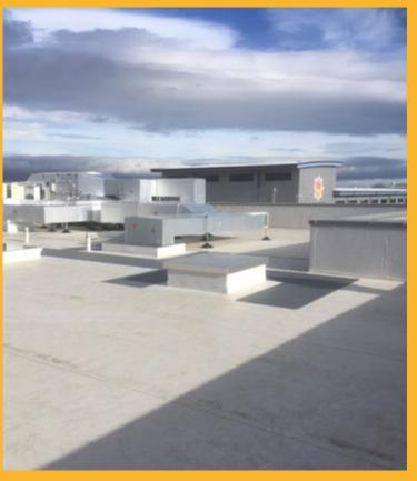
The reinforced PVC waterproof membrane offers a durable solution for warm and cold roof constructions. As well as supplying high tensile strength, Sika-Trocal® SGK provides outstanding weathering and excellent flexibility in cold temperatures, which along with its easy-fit benefits; make it the ideal membrane for exposed flat roofs.
