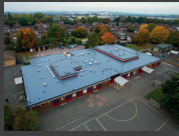
LIQUID APPLIED ROOFING
